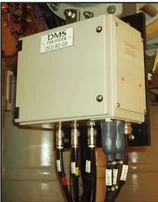
Each OCU takes the signal from a 3-phase set of sensors (couplers) and applies filtering to reject interference (noise) that can result from broadcast signals, discharges in nearby air-insulated equipment and other sources. The characteristic of the UHF pulse is then sent to the Equipment Cabinet.
