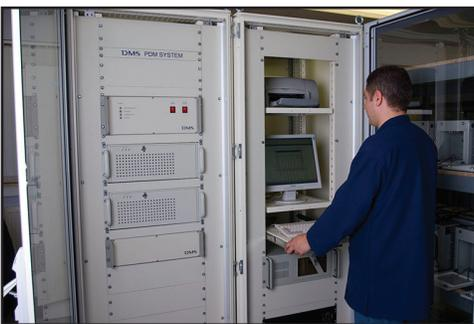
The Equipment Cabinet is typically located in the relay or control room and receives the optical data streams from the OCU's and transmits control signals back to the OCU (i.e. for the self test).
