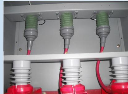
Iris Power EMCs are provided in coupler kits complete with all materials required for installation including the silicone rubber insulating boot.
