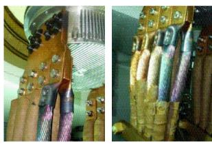
*Figure 4:* Crimped terminals and cables connected to the bushing's intermediate copper plate.
