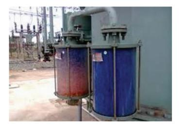
Liquid preservation systems limit the exposure of the transformer insulation structure to the atmosphere while allowing thermal expansion and contraction of the liquid due to load and ambient temperature variations. These liquid preservation systems are:
